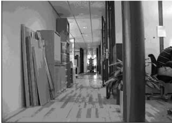
Figure 3.4: Telenor Headquarters: work zone.
